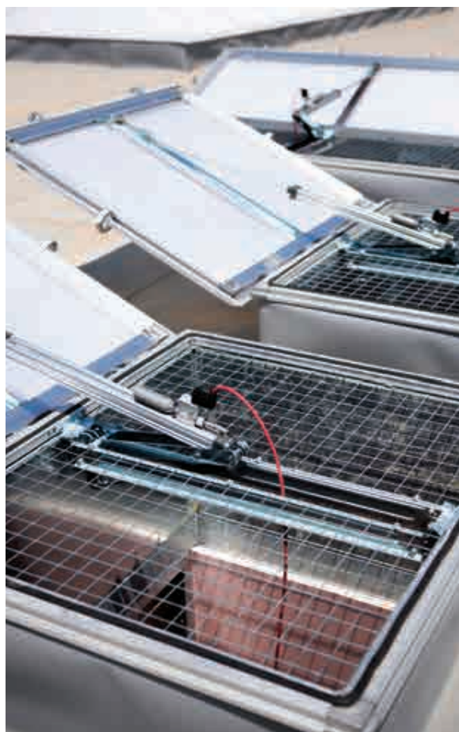
SMOKE OUT ® with pneumatic opening mechanism for maintenance
