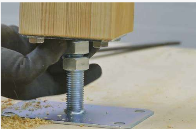
6 Overlaying the post on the threaded bar assembled with the bottom plate.
