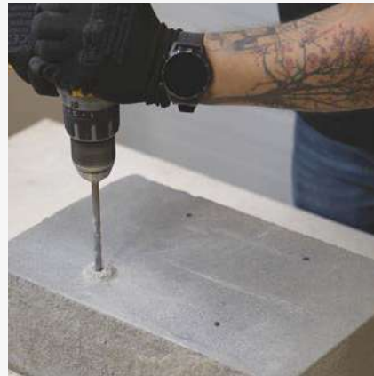
2 Reaming holes in concrete.
