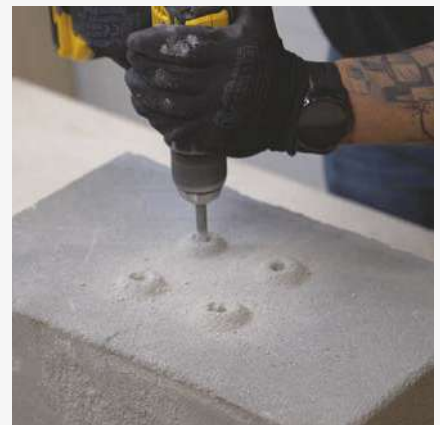
6 Reaming holes in concrete.
