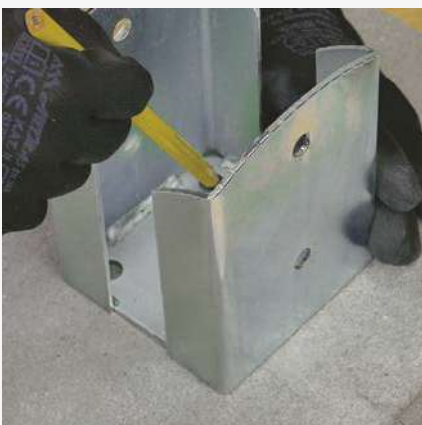
1 Determining hole locations.
