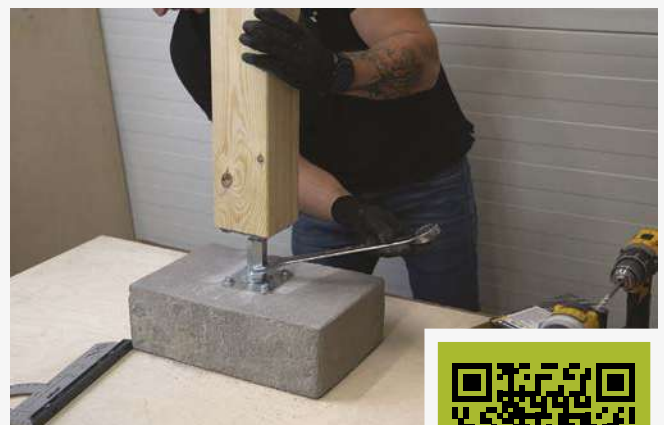
8 Adjusting the height of the post offset from the concrete.
