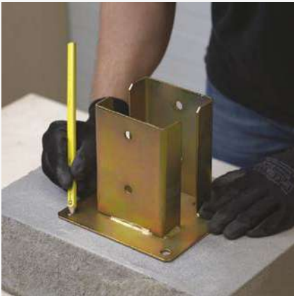
1 Determining hole locations for ring anchors.
