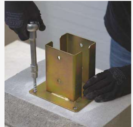
3 Fixing the support into concrete.
