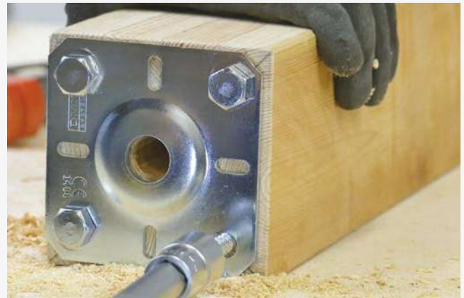
5 Fixing the top plate to the underside of the post.
