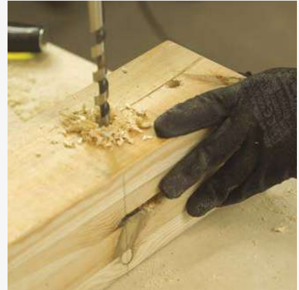
3 Drilling holes through.
