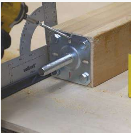
4 Additional bean holes for fully threaded screws, fixing at an angle of approximately 30°.
