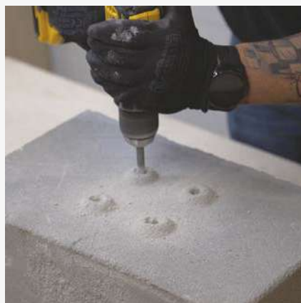
2 Reaming holes in concrete.
