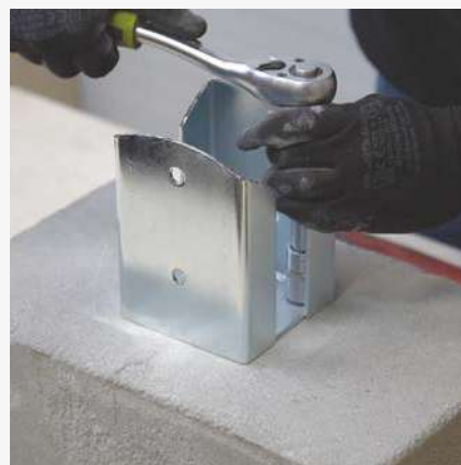
5 Fixing the support into concrete.
