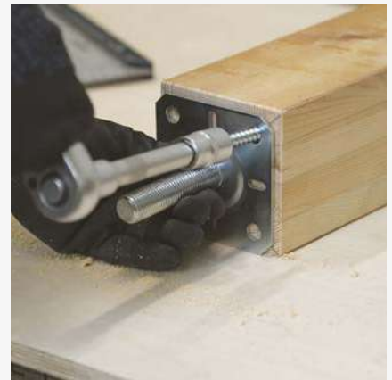
3 Fixing the top plate to the underside of the post.
