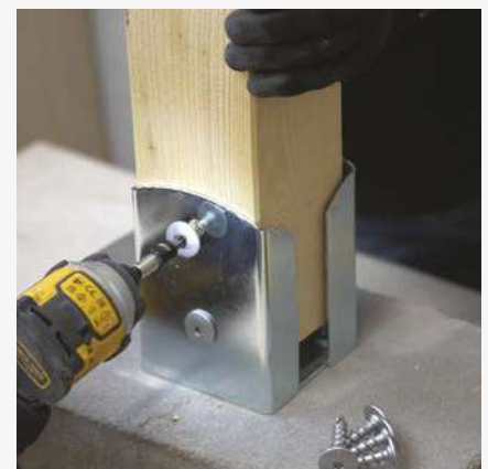
6 Setting the post into the support and screwing it into the garden structures.
