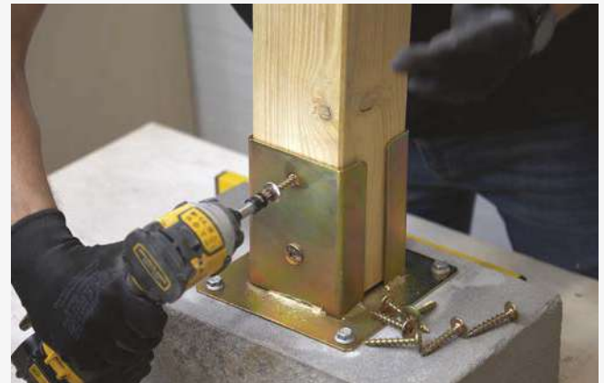
5 Screwing it into the garden structures.
