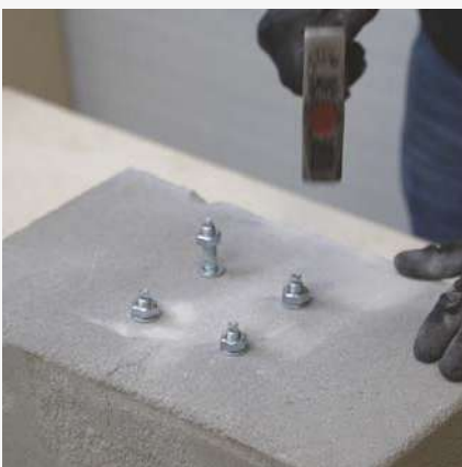
4 Driving in ring anchors.
